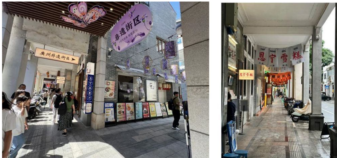
Figure 11. The continuous arcades along Enning Road clearly reveal the traditional “shop below, residence above” commercial residential layout. Source: Photograph by the author on October 21, 2024.
