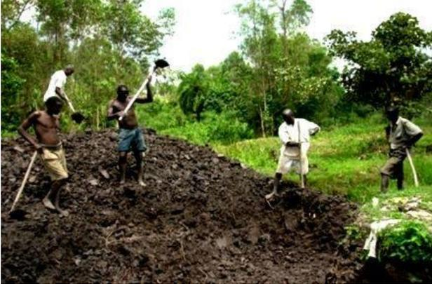
**Figure 3.** Extracting clay for making bricks and tiles.
