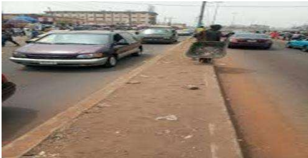
Figure 10. Road surface cover condition is being tarred. Source: Author's field survey, 2021.
