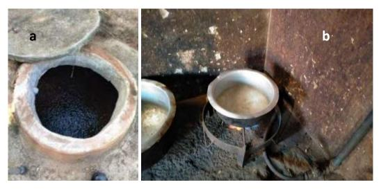
Figure 10. (a) Biogas digester. (b) Biogas stove.
